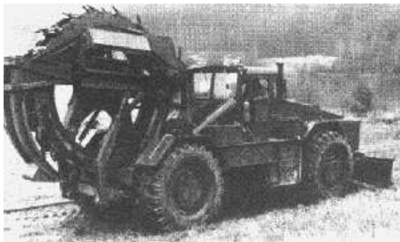
TMK-2 trenching machine (0/0/3)
